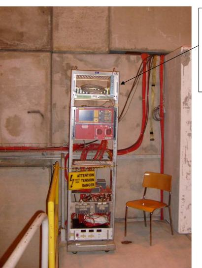
The high voltage system is just outside the radiation area.
